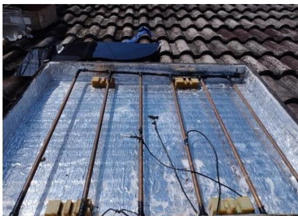
Figure 2. Copper pipe with evaporator chamber.
