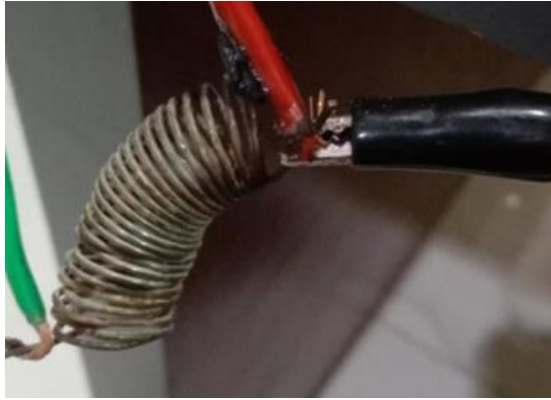
Figure 4. The heater coil mounted on the pipe.
